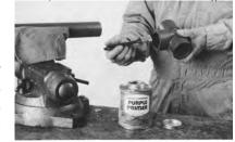
Apply again to the fitting socket. The second application is especially recommended for belled-end pipe and fittings fabricated from pipe stock, for many of them have especially hard inside-surfaces.
