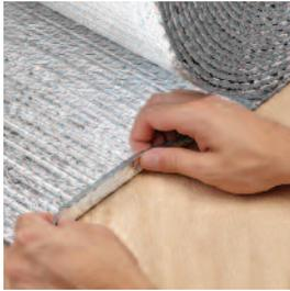
Product consists of two, 96% reflective layers of film bonded to two internal layers of heavy gauge polyethylene bubbles (5/16" thick). The product is available with a standard or staple tab edge (photo above). Reflectix offers their Reflective Insulation in 16", 24" and 48" widths by 25' and 100' lengths.
