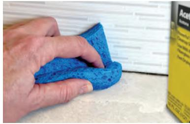
2. Apply **Acetone or Isopropyl Alcohol** to the silicone and let sit for a 1/2 hr or so before scrubbing the area with a scrubby sponge or brush. **Always use ventilation with any solvent cleaning solution.**
