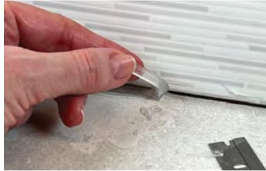
1. Cut away and remove all caulk with a caulk remover tool or razor blade.
