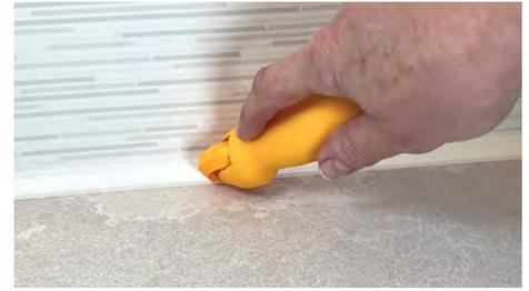
**MEASURE** – Lay the new trim strip along the application area to determine the length needed. Before cutting, add 1/8 inch. Cut with a razor blade or scissors.
