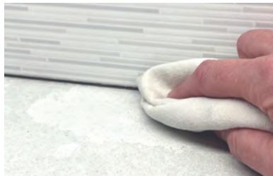
4. Thoroughly wipe down the area with **Acetone or Isopropyl Alcohol** to remove any silicone residue or sealant that is left behind.
