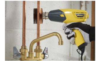
Thawing Pipes
