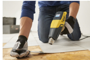
Removing Floor Tile
