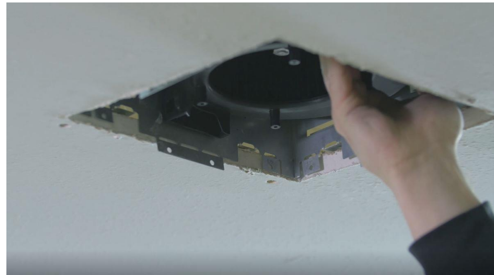
New construction Securing Tabs lock the fan into place
