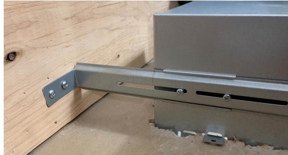
Joist hangers attach with screws to trusses or joists
