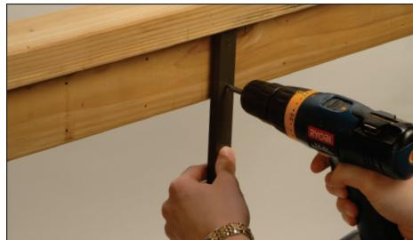
**Step 2:** The baluster spacing is 4-1/2" on-center and equal spacing for the end spacing. For posts set at 6' on-center, attach the first two balusters 2-1/4" on-center each side of the center line using four of the screws provided. Use the plastic washers when using treated lumber to prevent direct contact. Simply place the washer in between the rail and baluster.
