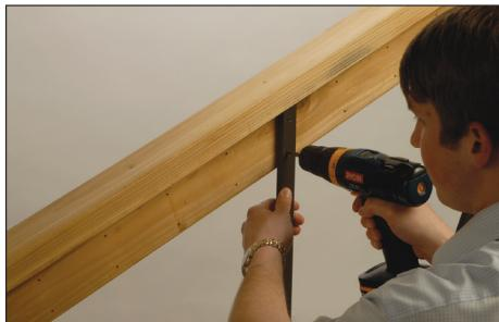
**Step 2:** The baluster spacing is 4-1/2" on-center and equal spacing for the end spacing. For posts set at 6' on-center, attach the first two balusters 2-1/4" on-center each side of the center line using four of the screws provided. Use the plastic washers when using treated lumber to prevent direct contact. Simply place the washer in between the rail and baluster.
