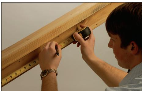
**Step 1:** Attach top and bottom stair rails to posts according to local building codes. The distance from the stair tread to the top of the rail is typically 36". Use a baluster as a guide to determine placement of the bottom rail. Find the center of the top and bottom rails and mark.
