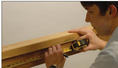
**Step 1:** Attach top and bottom rails to posts according to local building codes. The distance from the deck surface to the top of the rail is typically 36". Use a baluster as a guide to determine placement of the bottom rail. Find the center of the top and bottom rails and mark.
