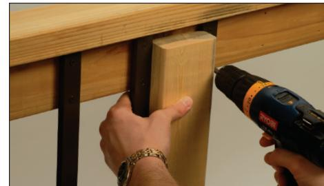
**Step 3:** Use a section of 2x4 to space the next baluster 3-1/2" from the first. Attach the rest of the balusters using the 2x4 as a spacer block. Cut two crush blocks from the wood or composite railing material you're using. Glue crush blocks to the bottom of the lower rail an equal distance from each post.
