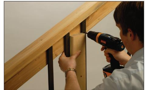
**Step 3:** Use a section of 2x4 to space the next baluster 3-1/2" from the first. Attach the rest of the balusters using the 2x4 as a spacer block.
