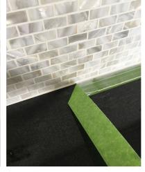
6. Seal the tiles and grout lines after grouting. We recommend using the DuPont™ StoneTech® Professional Sealer or 511 Impregnator to seal shell mosaic tile.
