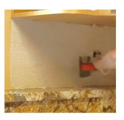
2) If to use the tile setting mat. Peel off the backing paper, place the mat in position and mark cuts if needed. Cut the mat with scissors or utility knife. Flatten air bubbles and creases. Cover all surfaces to be tiled. Cut a corner from the end of the mat to facilitate folding or corner. Set the tiles onto the mat evenly.
