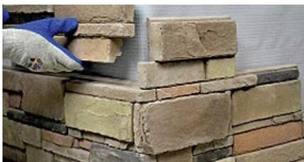
When inside and/or outside corners are present it is recommended that you start with inside corners first, then outside corners, then fill in between with flats. The first row locks onto the Starter Strip and the stones work better from left to right. When you get to the end of the each row measure and make the appropriate cut, using the remaining piece to begin your next row.
