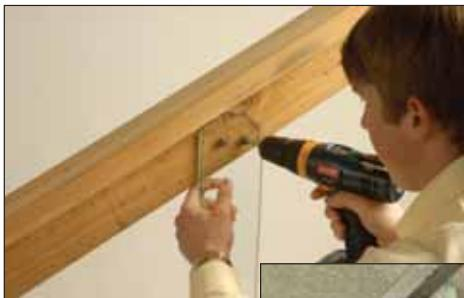
**Step 2:** Attach the first baluster on-center of the center line using four of the screws provided. Place screw cap in between rail and screw. Drive each screw until the rubber washer begins to mushroom. Do not over drive. Snap cap into place to conceal screw head.
