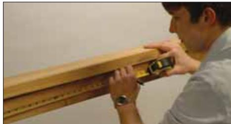
**Step 1:** Attach top and bottom rails to posts according to local building codes. The distance from the deck surface to the top of the rail is typically 36". Use a baluster as a guide to determine placement of the bottom rail. Find the center of the top and bottom rails and mark. Rail length  $\div 2$  = Center of Rail.
