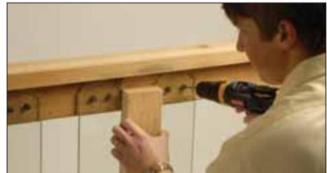
**Step 3:** Use a section of 2x4 to space the next baluster 3-1/2" from the first. Attach the rest of the balusters using the 2x4 as a spacer block. Cut two crush blocks from the wood or composite railing material you're using. Glue crush blocks to the bottom of the lower rail an equal distance from each post.
