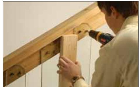
**Step 3:** Use a section of 2x4 to space the next baluster 3-1/2" from the first. Attach the rest of the balusters using the 2x4 as a spacer block.
