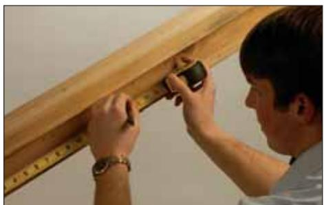
**Step 1:** Attach top and bottom stair rails to posts according to local building codes. The distance from the front edge of the stair tread to the top of the rail is typically 36". Use a baluster as a guide to determine placement of the bottom rail. Find the center of the top and bottom rails and mark.
