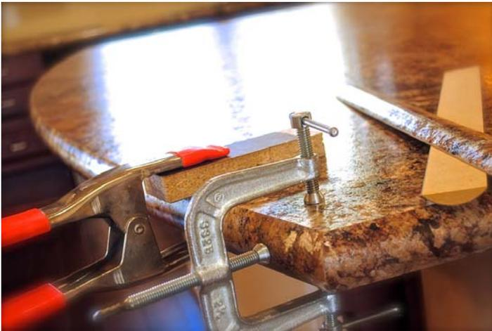
Move the block and clamp to each taping location during the taping process to secure a flush application. Twist one end of your tape to make removal easier.
