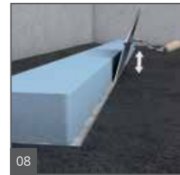
08 Apply thinset mortar to support the profile at desired height.
