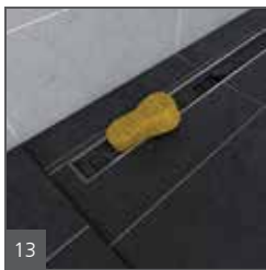
13 Clean off any excess grout.
