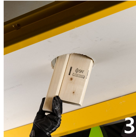
3 Using a rotary tool, cut a six-inch round hole through the ceiling (only if required). Insert 2x4 wood supports into the ceiling. 2x4s will be used to create a ceiling support system to secure the island hood where studs are not available.
