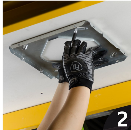
2 Take the included ceiling plate and mark the location by tracing along the inside.
