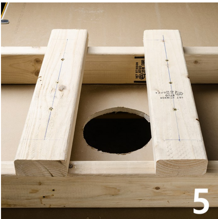
5 The T-shaped 2x4s should align and meet above the holes for the ceiling plate.
