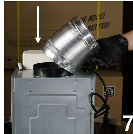
7 Connect the included duct pipe to the air damper.
