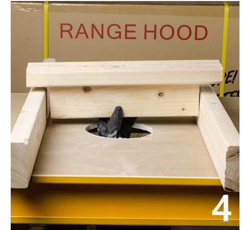
4 Arrange the 2x4s as shown. Two L-shaped pieces should be placed across from each other. T-shaped pieces are added next to form a square base around the perimeter of the exhaust hole. You may need roof access.
