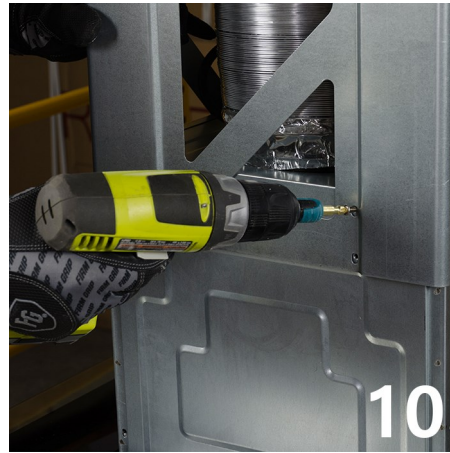
Take the smaller lower support frame and fasten it to the range hood main unit with the included screws.
