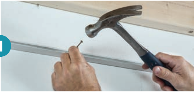
Install wall molding
