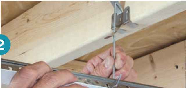
Suspend main beams with hanger wire or QuickHang™ hardware* (shown above: QuickHang hooks and brackets)
