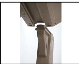
Slide mailbox post section over treated pine 4" x 4" post (make sure mounting arm is facing the street) Choose desired location of mailbox and install 48" long 4x4 treated pine post into the ground (16" into the ground and 32" remaining above ground)
