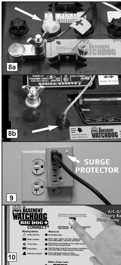
Simply insert the fluid sensor in the top of the battery next to the arrow.
