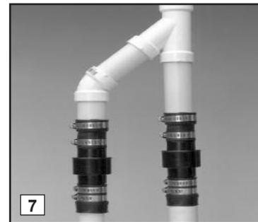
7. Connect a piece of 1½" PVC pipe above the check valve of the Basement Watchdog pump, and attach a 45° elbow to that pipe. Extend another piece of pipe to reach from the 45° elbow to the "Y" connector on the other pipe.
