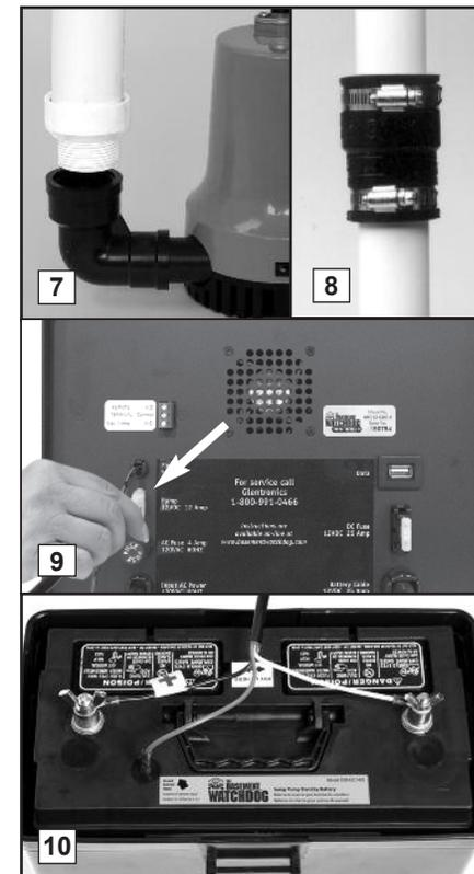
10. Replace the fluid sensor in the top of the battery. Connect the battery cables to the battery...the WHITE wire to the NEGATIVE (-) post, and then the BLACK wire to the POSITIVE (+) post. Tighten the wing nuts. Replace the fluid sensor.
