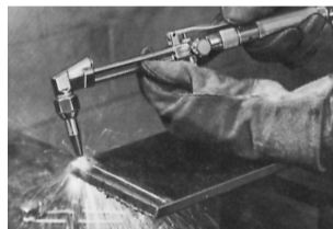
Figure 19. Steel Flame Cutting
