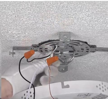
Step 5: Remove the hook
