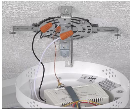
Step 4: Match up the wires
