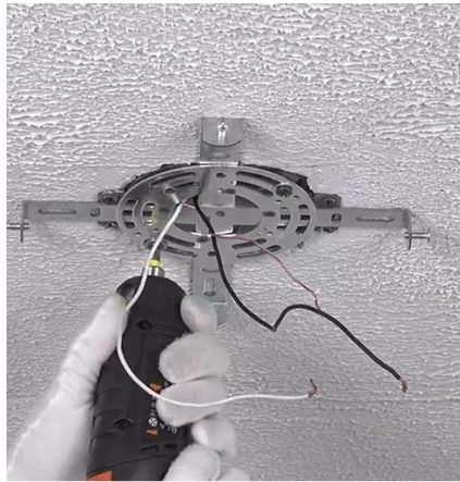
Step 1: Mount the Bracket
