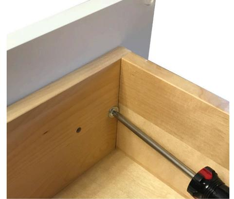
2 If additional adjustment is required, loosen screws and twist drawer front for proper alignment. Tighten screws securely.
