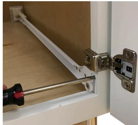
3 Attach runner to inside edge of face frame. Note the roller wheel is positioned at the bottom with the opening up. Repeat on opposite side.
