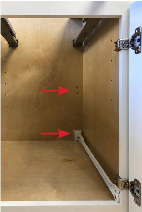
In a standard Base Cabinet there are two locations a Roll-out Tray can be installed, indicated by the two sets of pre-drilled holes on the back panel.
