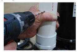
3. Measure 6 inches up as show in image. Drill a 1/4"\* anti-airlock hole into PVC pipe.
