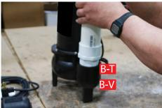
1. Attach PVC pipe (G) to coupling (H) using PVC pipe primer\* and glue\*. Push down to secure.
