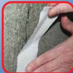
3. PRESS FIRMLY INTO PLACE
