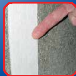
4. SEAM TAPE IS READY TO COAT
