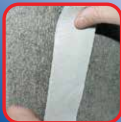
2. LINE TAPE UP WITH SEAM
