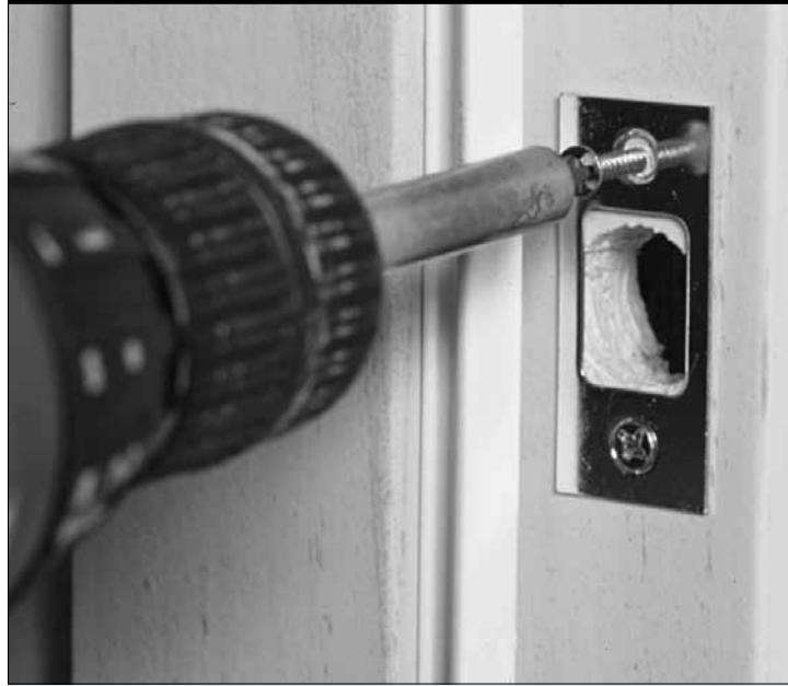
FIGURE 22: Screws fasten the latch plate to the door slab.
