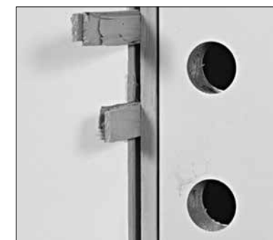
FIGURE 12: Shims are placed above and below the dead bolt hole (points G in figure 10).
