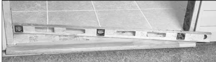
FIGURE 1: A clean, level, solid sub-floor area is essential for successful installation.
