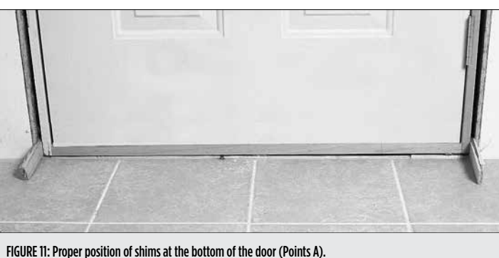
FIGURE 11: Proper position of shims at the bottom of the door (Points A).
