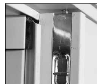
FIGURE 14: Correct sagging until the flush bolt slides freely into the pre-drilled hole (not typical of most units) in the head/threshold.
