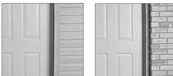
FIGURES 6 and 7: The exterior trim (brickmould) rests up against exterior sheathing or slides into the opening of exterior brick.
