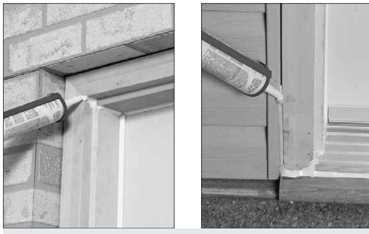
FIGURES 26 and 27: Caulk the jambs and the exterior trim.
