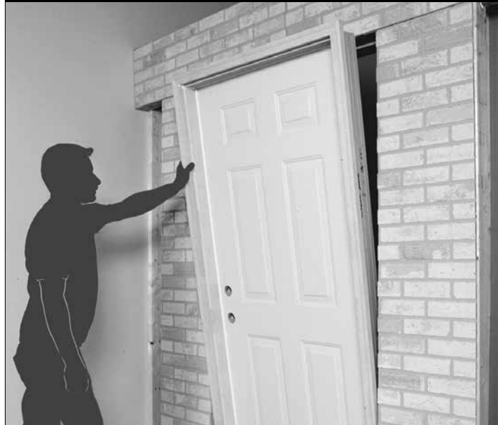
FIGURE 5: Place the sill in the opening first and then tilt the door up into the opening.
