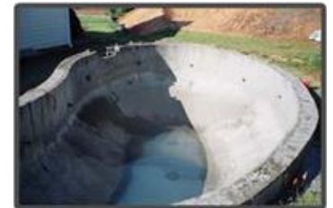
1. Prepare the Surface
