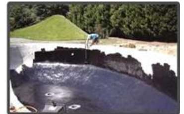
2. Apply the Coating
