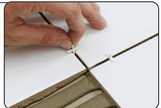
The QEP® Traditional Flexible Tile Spacers maintain consistent grout joints and align tiles when installing floor or wall tiles. These spacers are made from flexible plastic, which allows for slight compression as needed during tile installation. Reusable and compatible with various tile types, these spacers are imperative to keep on hand for professional looking results.
