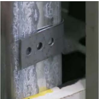
Ear of wood stud anchor
