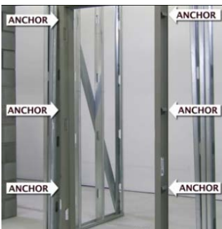
Proper anchor spacing
