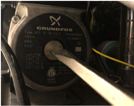
Figure 54 - Bleeding the Internal Pump
