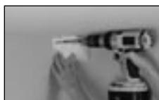
**Option #1** - Using Focal Point corner blocks: drill a 3/16" hole in center of each tab on the blocks. Install corner blocks in each corner and connector blocks in the center of each wall. Install blocks prior to installing the Quick Clips. Use polyurethane adhesive between mouldings and blocks.
