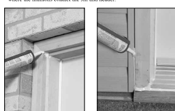
Figures 31 and 32: Caulk the jamb and the exterior rim.
