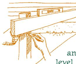
Transfer the joist hanger height to the posts using a joist and level, or by using string and a line level.
