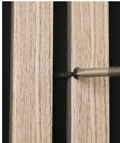
STEP 5: Fix with screws
