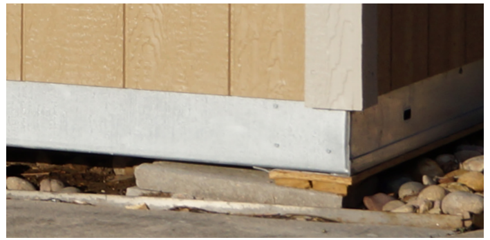
Figure 2 - Close-up of leveling with blocks & shims
