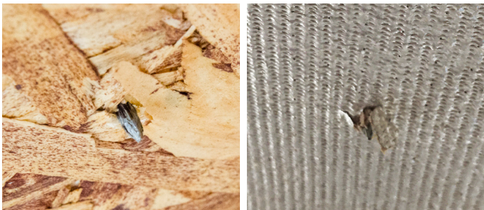
Roofing nails piercing roof decking
