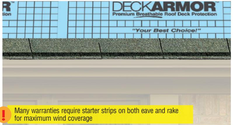
**!** Many warranties require starter strips on both eave and rake for maximum wind coverage
