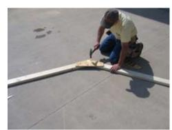
Install the truss gussets as shown and secure with 2" nails.
