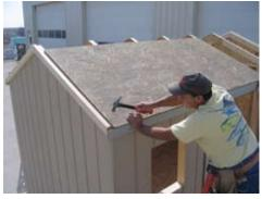
Next install roof sheeting as shown and fasten with 2" nails.
