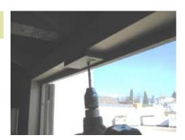
Drill a 5/16" hole for the barrel bolt.
