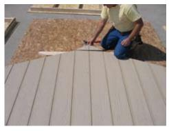
Make sure the small piece of Smart side is installed at the top.
