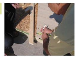
Measure 2" for rakes as shown at the bottom.
