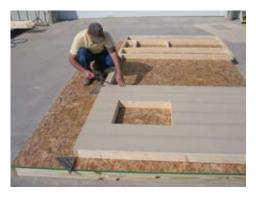
Next make sure top is flush with 2x4 and fasten with 2" nails.
