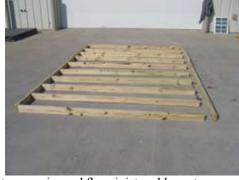
Locate your rim and floor joist and layout as shown.
