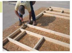
Install the 2x4 header and fasten with 3" nails.
