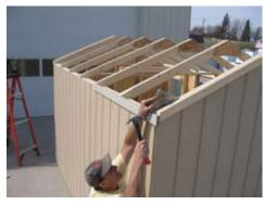
Install 2 3/4" trim as shown, keep flush with the outside of the rake and fasten with 2" nails.
