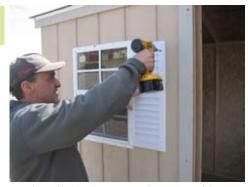
Next install the shutters and secure with provided screws for shutters.
