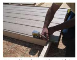
Install Smartside as shown. Make sure it is 3" to the bottom of the 2x4.
