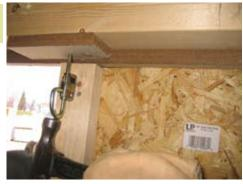
Use the hammer again to tap on the barrel bolt to locate where to drill your 5/16" hole.
