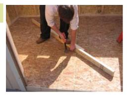
Fasten bracing temporarily with 2 1/2" screws.
