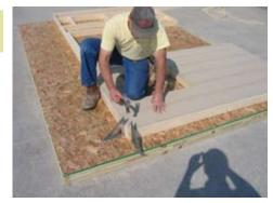
Make sure the corners are flush as shown and fasten with 2" nails.
