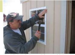
Next install the window and fasten with 2" nails as shown.
