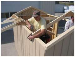
Install the truss as shown and fasten with 3" nails.
