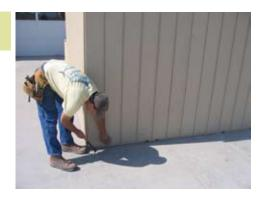
Next nail the bottom of the building with 2" nails 8" o.c all the way around.
