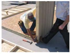
Make sure the wall is flush on the end and put pressue on the outside as shown, fasten with 3" nails.
