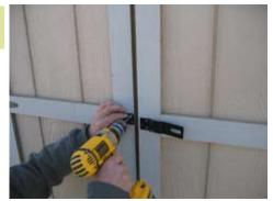
Now install the latch on the door, with 1 1/4" screws.
