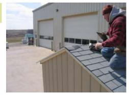
Cut the ridge caps and install the first one as shown.
