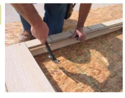
Next install door stops as shown. Keep flush with the top of 2x4 not Smartside and secure with 2" nails.
