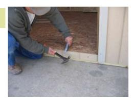
Locate 3" Smartside siding pieces and keep flush with the top of the floor and secure with 2" nails.
