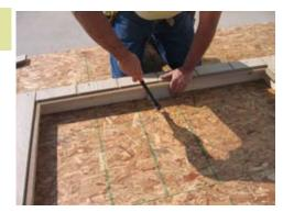
Install the trim block in the center of the header and secure with 2" nails.
