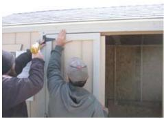
Install the door with 1 1/4" black headed screws, 3 per hinge, as well as (1) 2 1/3" blackheaded screw per hinge.
