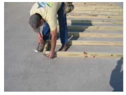
Start at the corner and use the square to make sure the corner is flush and fasten with 3" nails.
