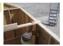
Measure your wall before fastening the last brace with 2 1/2" screws.
