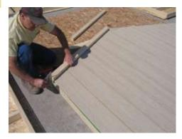
Keep the rake flush at the bottom and secure with 3" nails.
