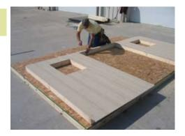
Fasten header piece with 2" nails as shown in picture before.
