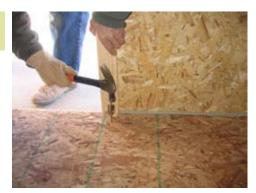
Use the hammer to tap on the barrel bolt to locate where to drill your 5/6" hole.
