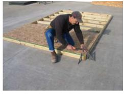
Make sure the OSB is flush with the 2x4 and fasten with 2" nails.
