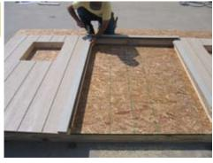
Install the 2 3/4" trim around the door and secure with 2" nails.
