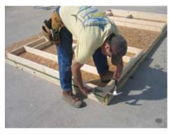
Fasten the wall with 3" nails as shown.
