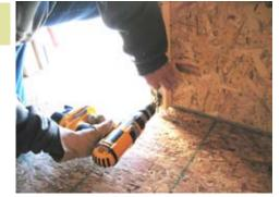
Install the barrel bolts as shown with 1 1/4" screws.
