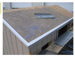
Measure 6" over the drip edge and snap a chalk line as shown for starter strips.
