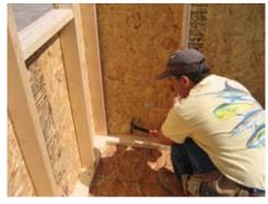
Make sure the walls are in place, and secure with 3" nails.
