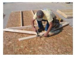
Fasten the truss with 3" nails as shown.
