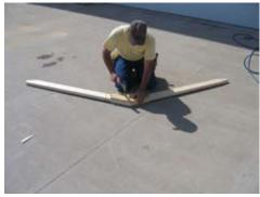
Flip the truss around and do the same with the gusset.
