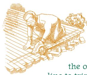
When all of the decking has been secured, remove the bumper board from the side joist and snap a chalk line across the decking on the other side. Use this chalk line to trim the decking boards flush with the side joist. Use a circular saw for this task and adjust the blade depth to cut just the decking, not the side joist. Apply end-cut solution to all cut ends.
