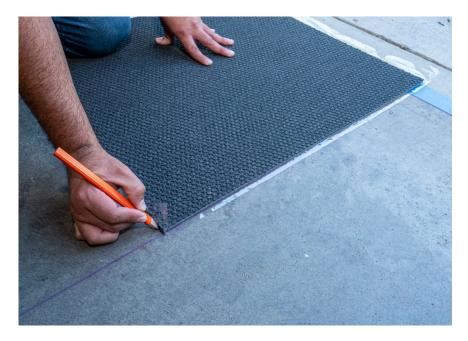
Before plastic backing is removed, place tile 1" over painters tape. Mark the back of your tile. The intersection of the center line and the line on the back of the tile will be your starting point.
