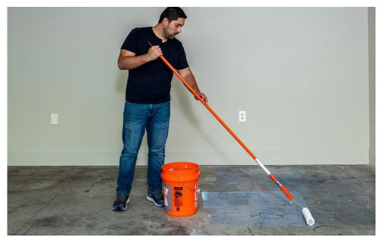
Pour LifeTiles<sup>®</sup> Primer into bucket. Do not dilute. Apply to floor using 3/8" nap or foam roller from back to front of garage. Be sure to include under the transition strip. Do not puddle. Additional coats may be required upon visual inspection over extremely porous concrete. Allow primer to dry to the touch.
