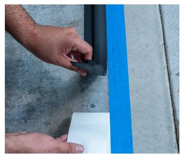
· Remove the tape backing and line the transition strip next to the painters tape.
